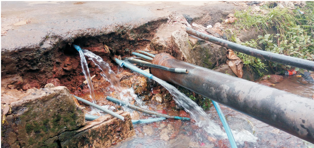
Destroyed water pipes along the Kissy Bye Pass Road Freetown
